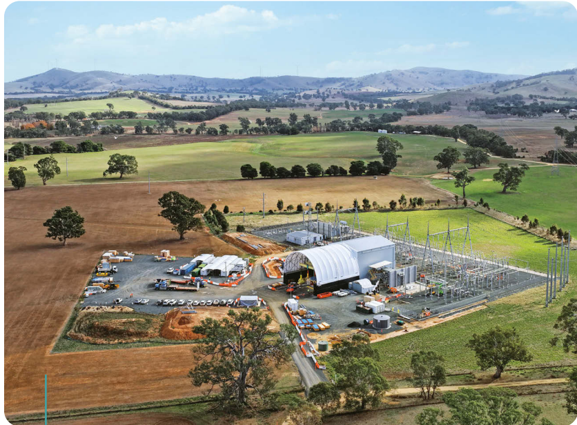
Beon Energy Solutions, VPN's engineering, procurement and construction services arm, constructed Australia's largest synchronous condenser at Ararat Terminal Station, helping stabilise the electricity grid and enable up to 600 MW of new renewable generation in Western Victoria.
